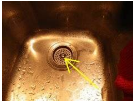
Photo 48-2 Sink stopper is defective and doesn't seem to hold water when tested.
