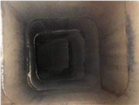
Photo 41-3 Second chimney flue appears to be okay.
