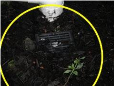
Photo 5-1 Grate to close to foundation and is allowing water to pool next to foundation where water appears to be coming in basement.
